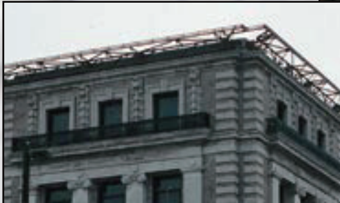
This heritage building gets a completed restoration with custom cresting.
