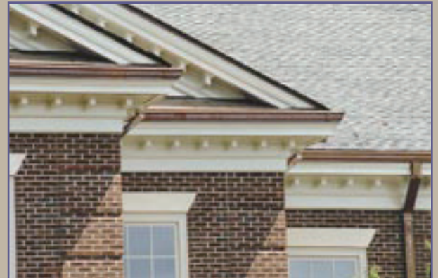
Photo above illustrates the use of custom crown mouldings and dentils.
